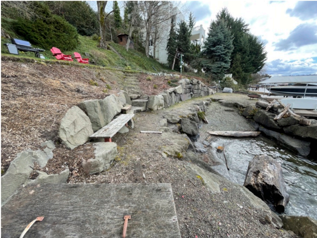
Photo 3 - Rock retaining wall to be moved away from shore.
