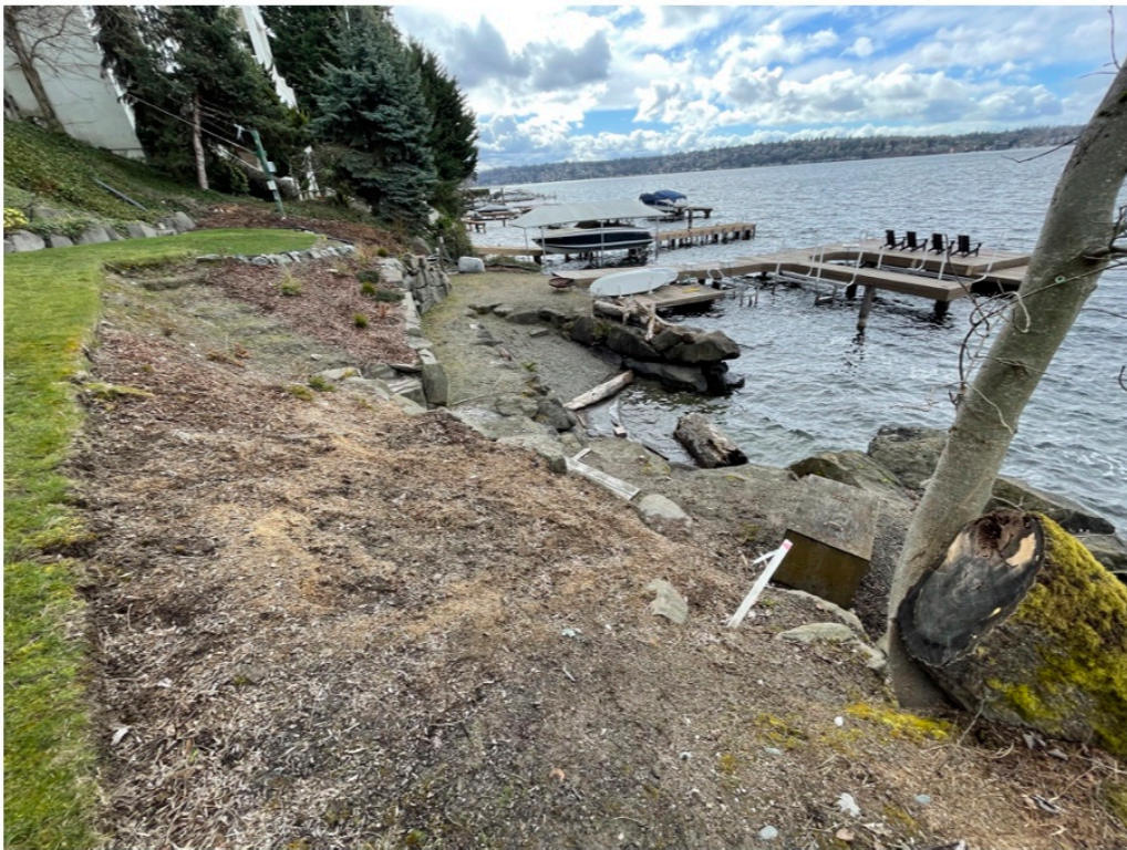
Photo 4 - Top of retaining wall to be relocated away from shore.
